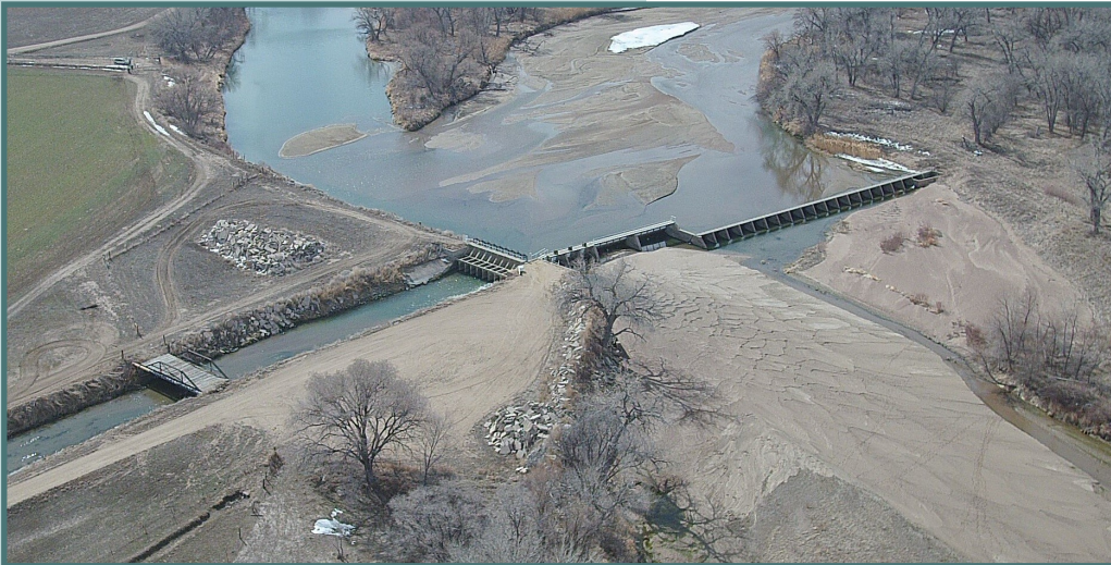
Prewitt Diversion Dam, March 14, 2023, Colorado
