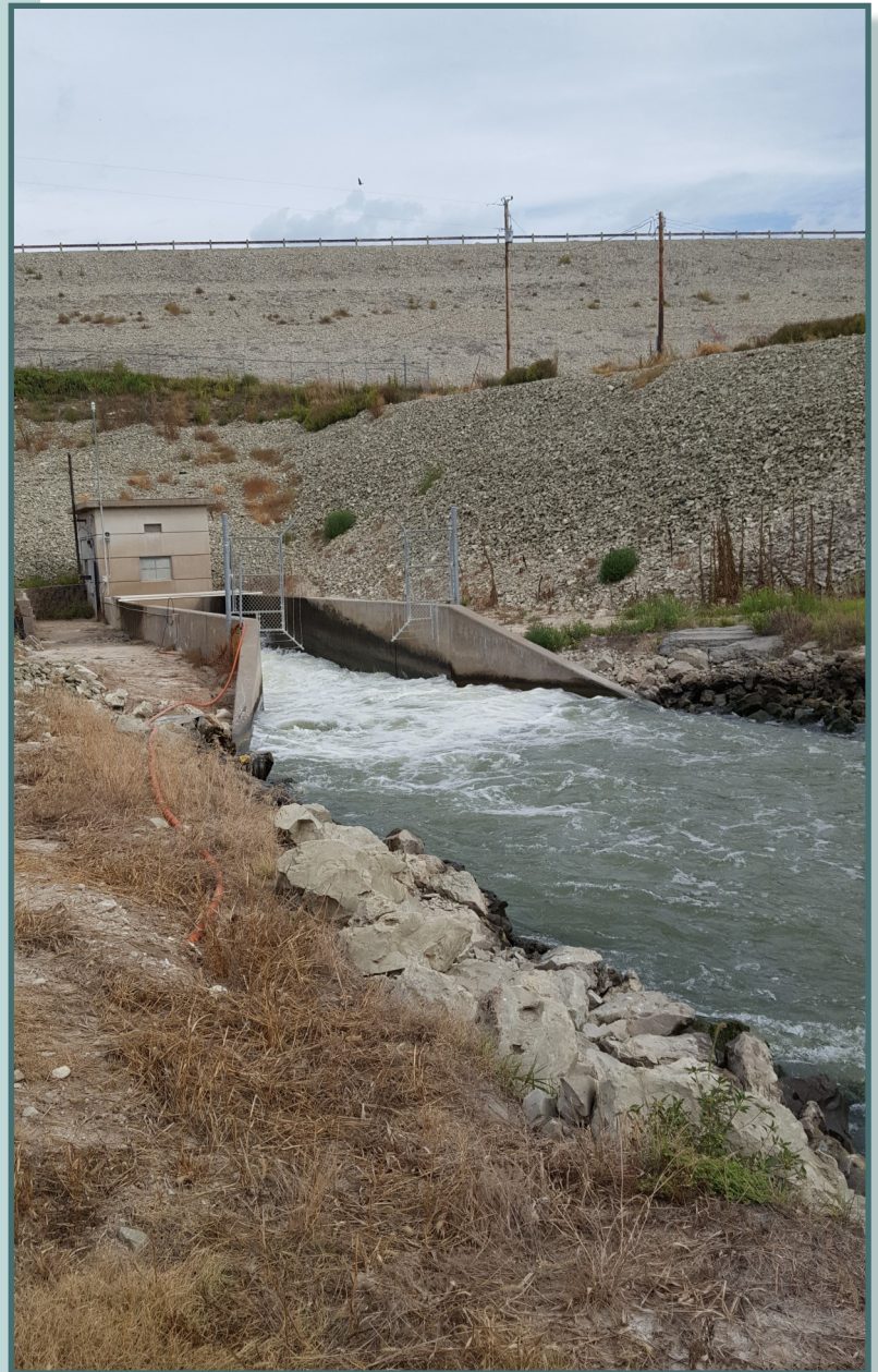
Outlet at Medicine Creek Dam.
