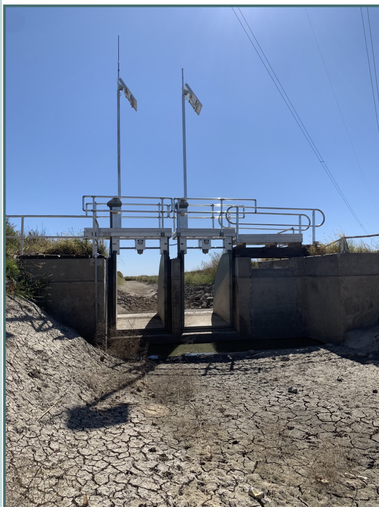
Back view of the newly installed control gates on Meeker Canal.
