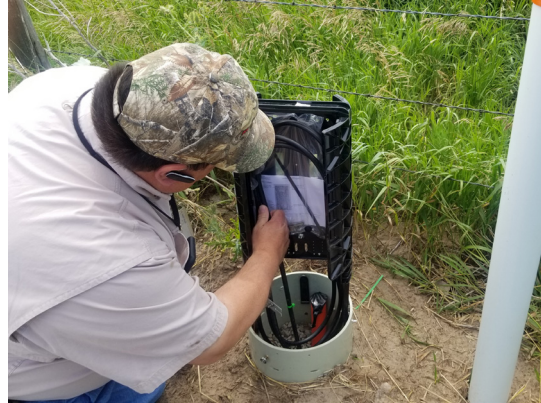
Technician checking pedestal on new fiber project. Photo Credit: Mary Ridder
