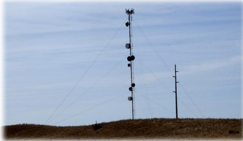
Cell tower-Highway 2-East of Dunning
