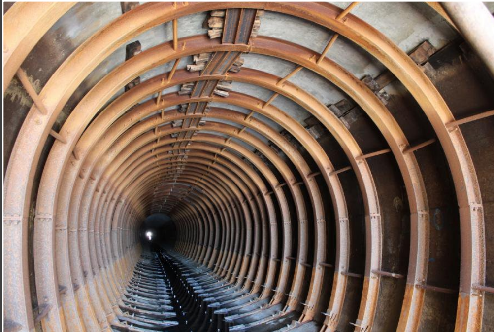
Gering/Ft. Laramie Tunnel repairs
