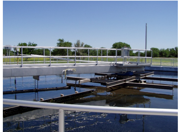
This photo shows a Wastewater Treatment Facility for Lincoln.
