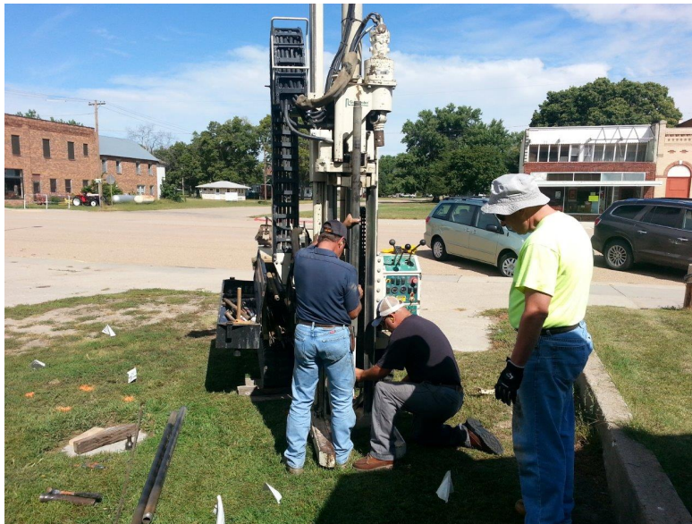
Direct push technology collecting soil or groundwater samples
