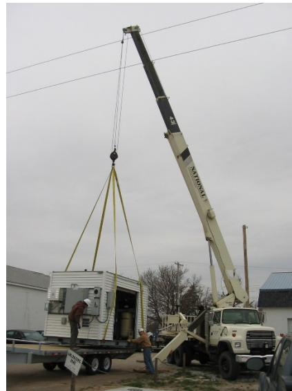
Moving a surplus remediation system
