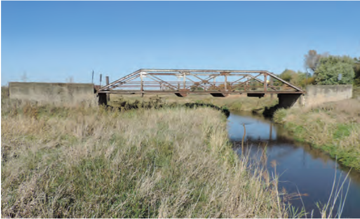
County Bridge Match Program Project North of Creighton ( Before )
