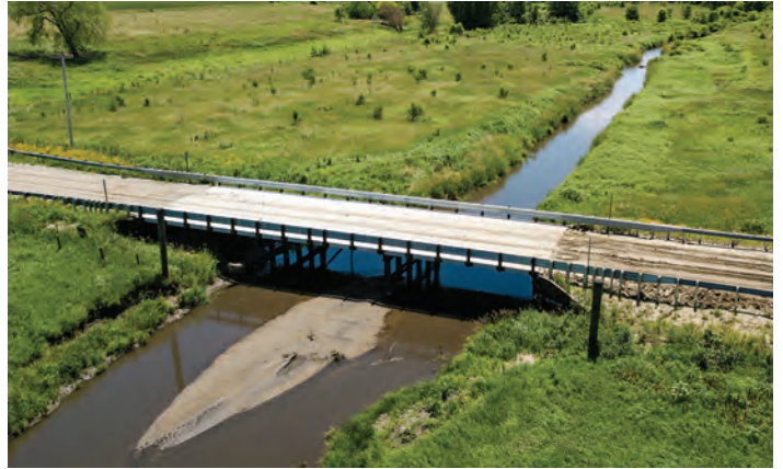
County Bridge Match Program Project North of Creighton ( After )
