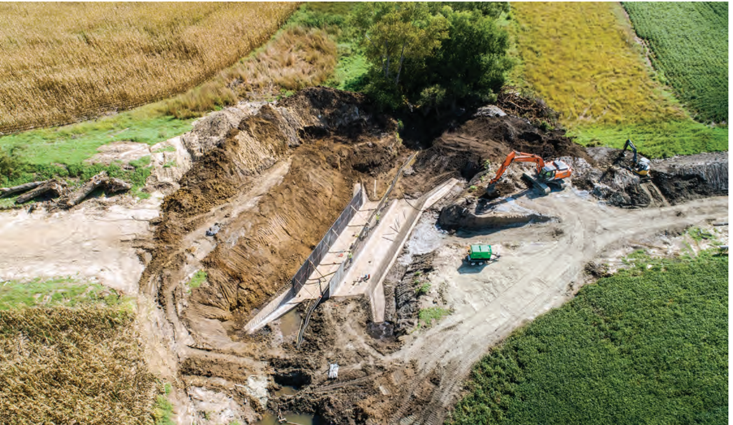
County Bridge Construction Site West of Palmyra
