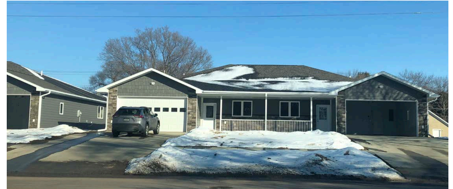
Newly-built rental units in Bloomfield.
