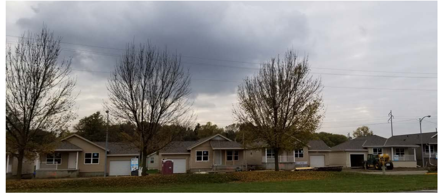
Habitat for Humanity of Omaha, new single-family ownership units.
