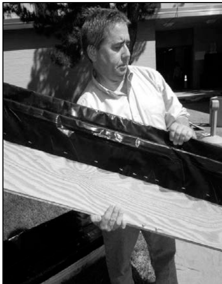
Figure 3-21. How to Hold a Chute for the Pour.
