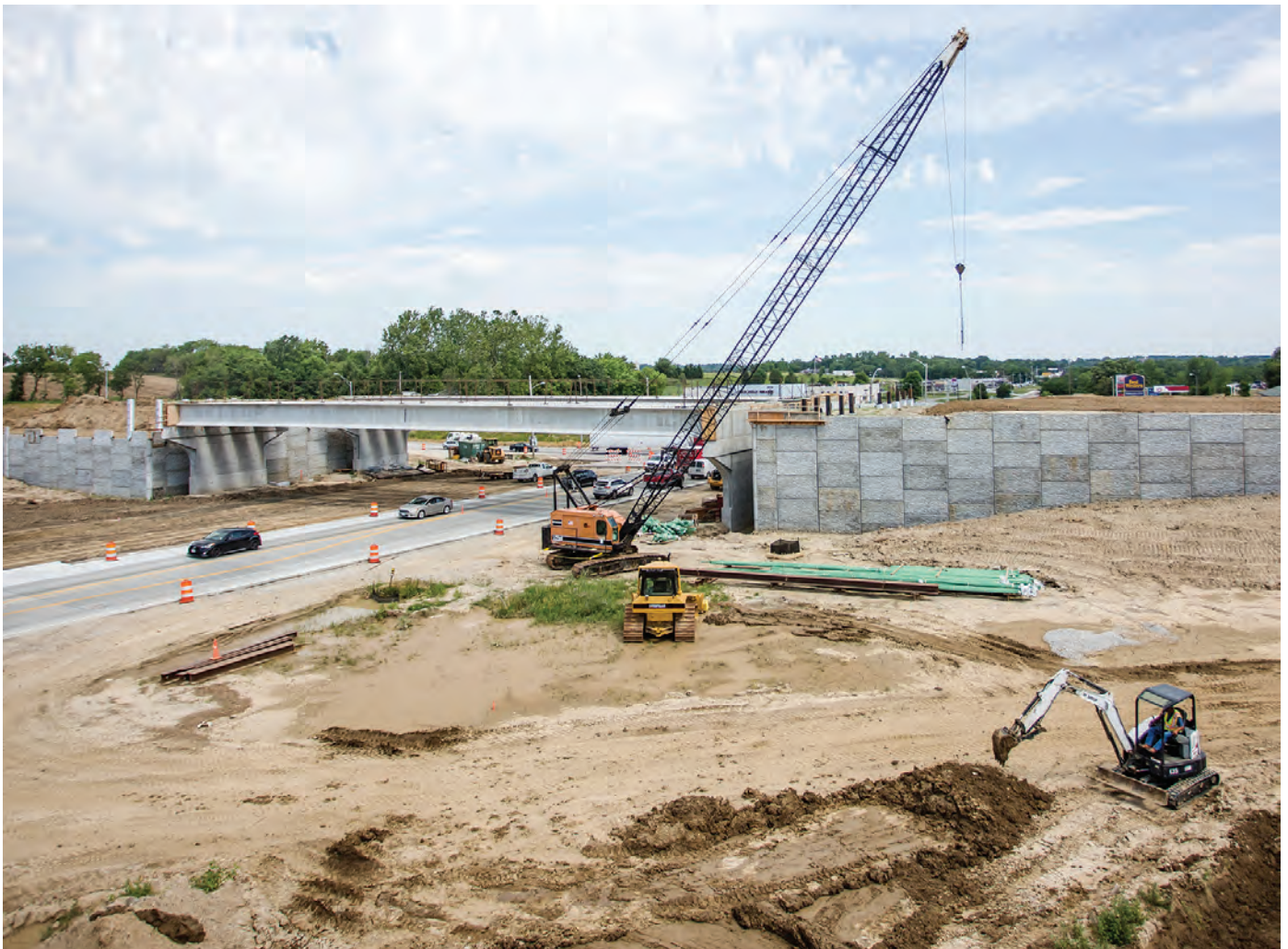
Construction on the Nebraska City project.
