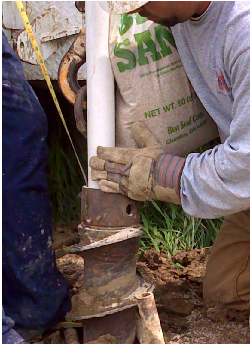
Installing a monitoring well near Clearwater, NE.
