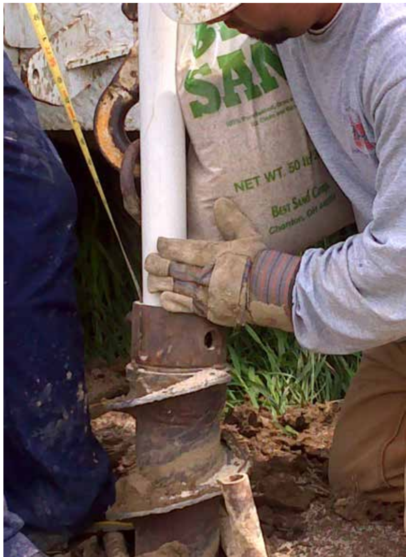
Installing a monitoring well near Clearwater, NE.
