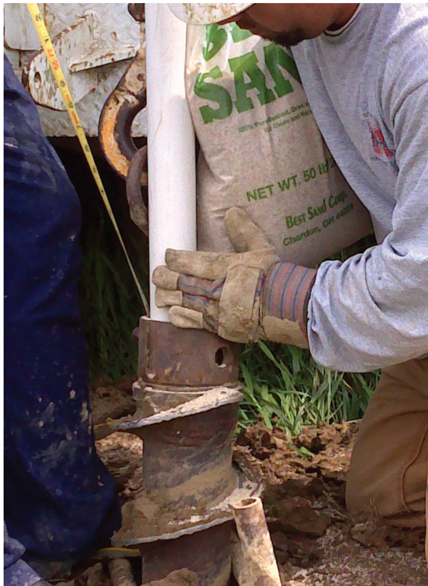
Installing a monitoring well near Clearwater, NE.
