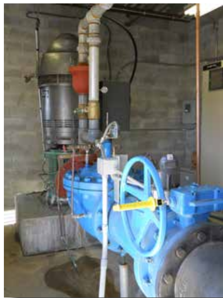
Public Water Supply well capable of pumping thousands of gallons per minute (Hastings, NE).
