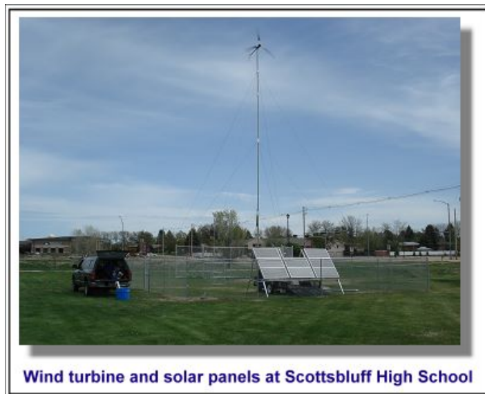
Renewable Energy – The wind and sun power the NDEQ air quality monitoring station in Scottsbluff, NE. Courtesy, Scottsbluff Star Herald.
