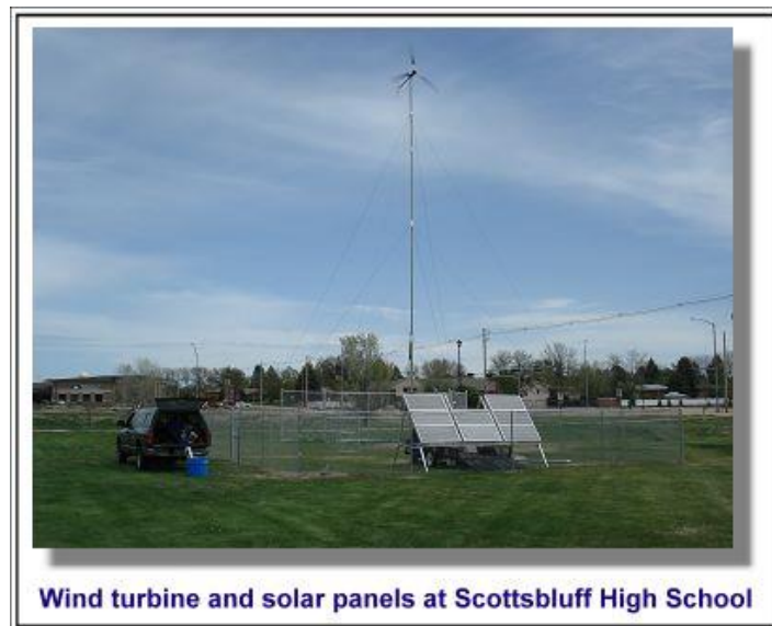
Renewable Energy – The wind and sun power the NDEQ air quality monitoring station in Scottsbluff, NE. Courtesy, Scottsbluff Star Herald.
