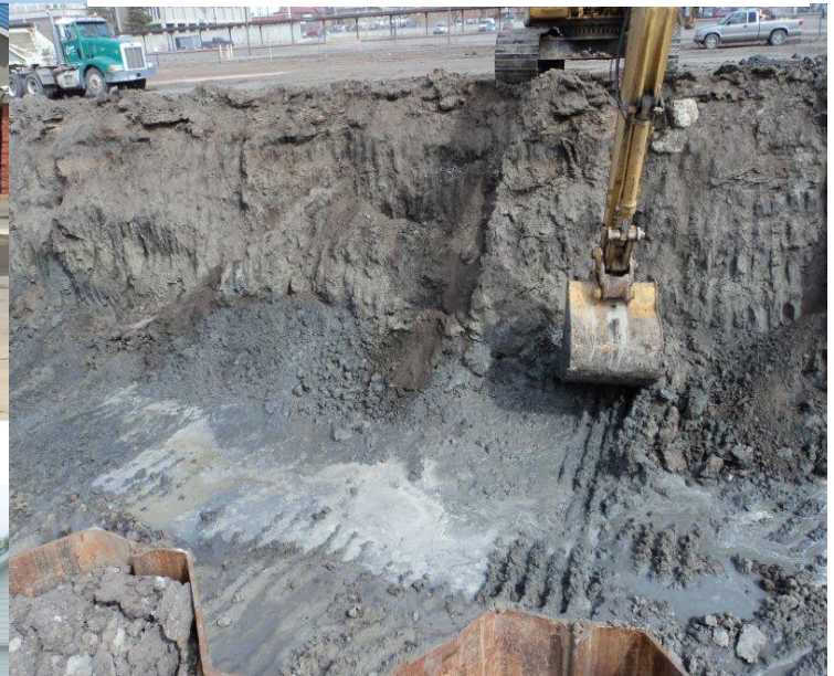
Pictured at left is an auger drill rig installing a monitor well during a Tier 1 site assessment. Below, right: Excavation of diesel fuel-contaminated soil (gray-green) and removal of free product (liquid) as part of a major redevelopment project. Below, left: A typical equipment trailer used to remove gasoline vapors from the subsurface soil and remediate ground water contamination.
