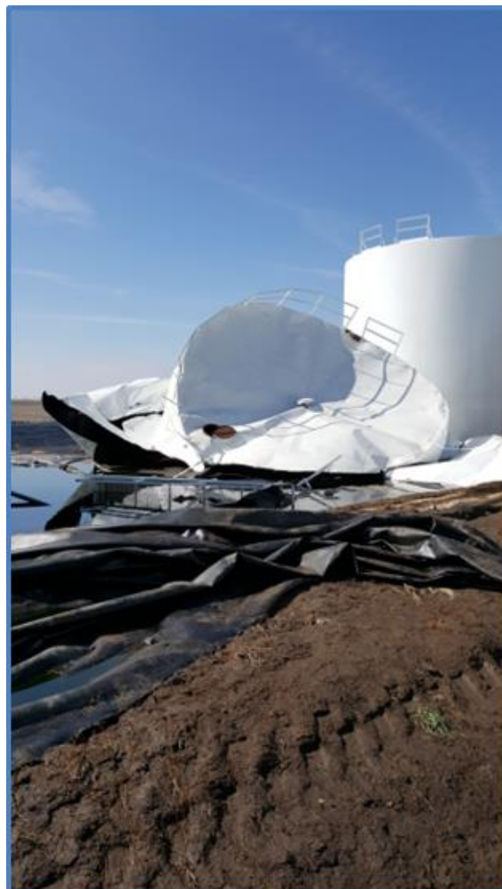
On March 2 nd there was a catastrophic failure of a liquid fertilizer tank at a Dorchester Coop facility. Approximately 165,000 gallons of product was released. See page 94 for more information about NDEQ Emergency Response efforts.
