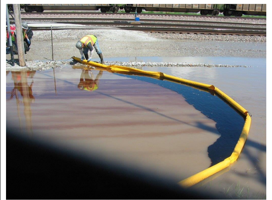
NDEQ Emergency Response Team members helped deploy oil containment booms to control releases associated with heavy rains at Burlington Northern's Hobson Yard in May, 2015. See page 94 for more information about NDEQ Emergency Response efforts.
