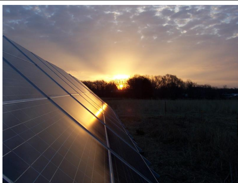
This solar-powered monitor near Weeping Water, is one of two NDEQ air monitoring sites that are powered totally through renewable energy sources. See page 26 for more information.
