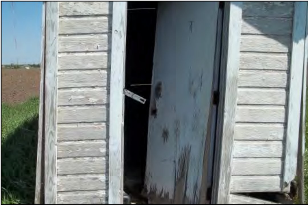
Shed with entrance to a storm cellar
