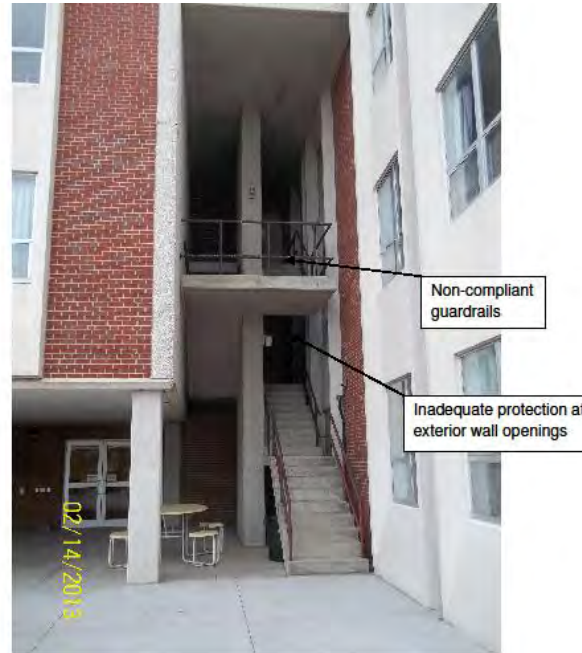
Phillips Addition Outside Stair
