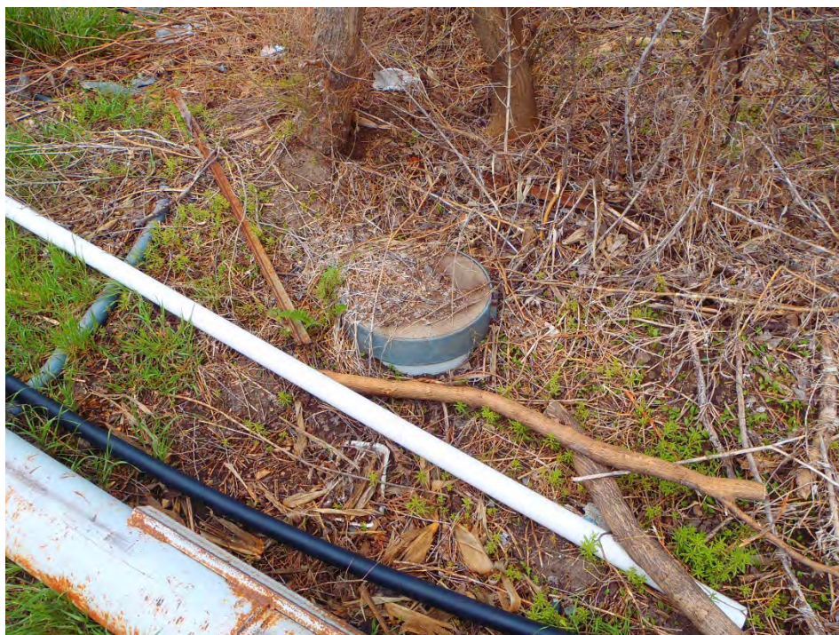
Photo10: Small manhole noted near the irrigation well in Photo 9. The function of the manhole was not evident.
