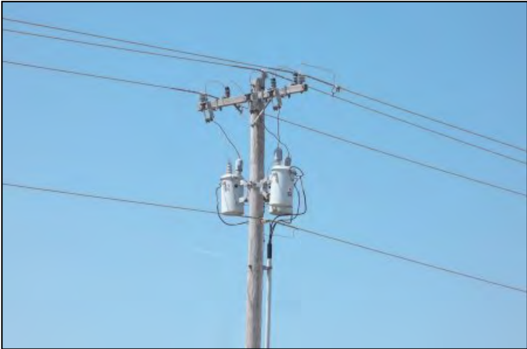
Pole-mounted transformers
