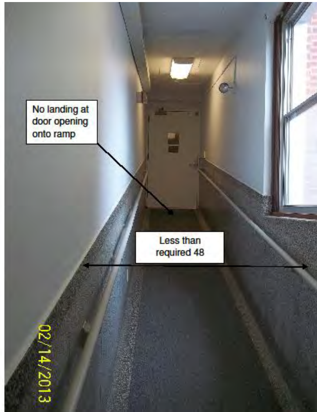
Administration Building Egress Ramp
