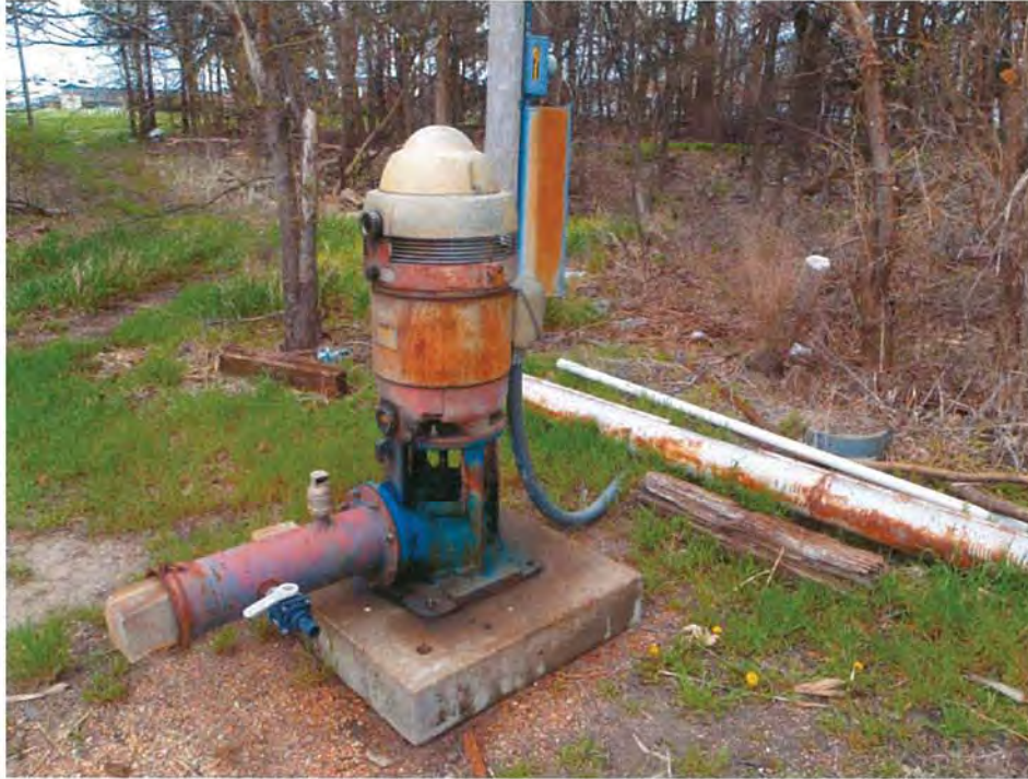
Photo 9: Second of two irrigation wells located on the assessment property. This well is located along the east boundary of the assessment property and is also electrically powered.
