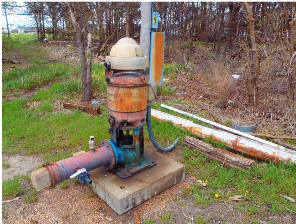
Photo 9: Second of two irrigation wells located on the assessment property. This well is located along the east boundary of the assessment property and is also electrically powered.
