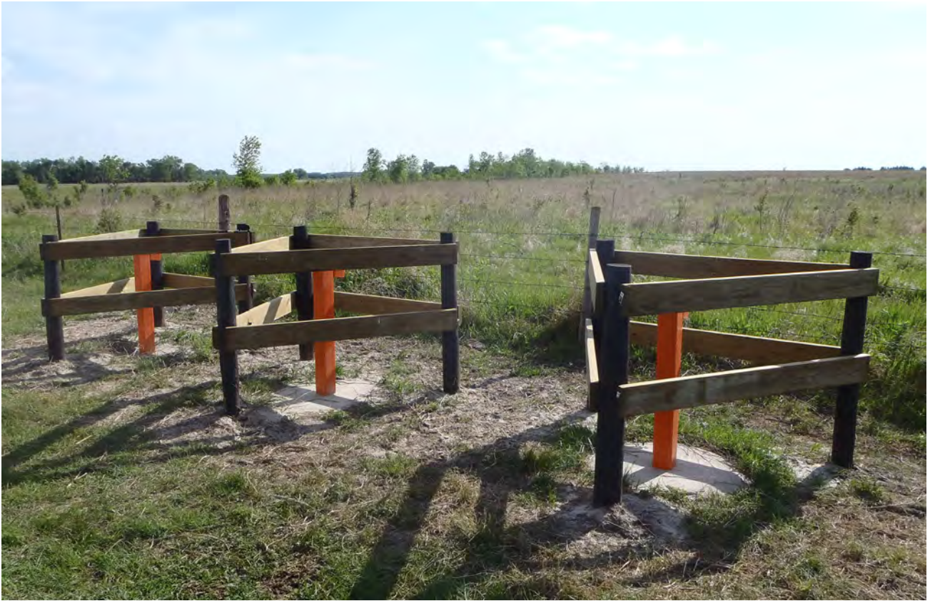
Dedicated monitoring wells in the Lower Loup Natural Resources District.
