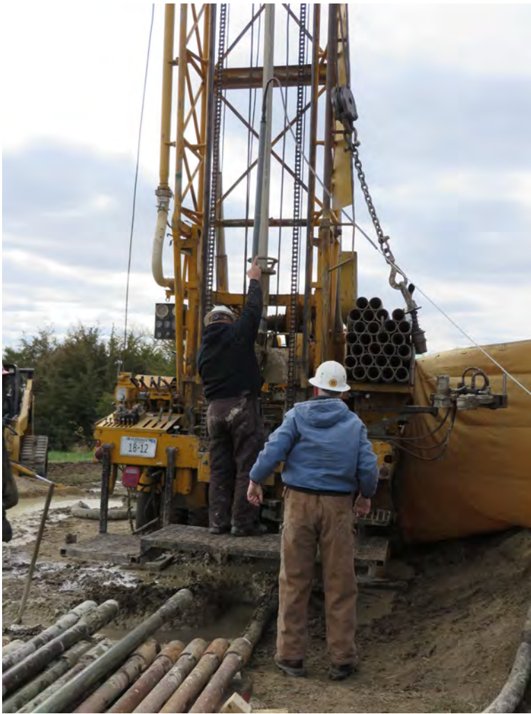
University of Nebraska Conservation and Survey Division drilling test holes in the Lower Loup Natural Resources District.
