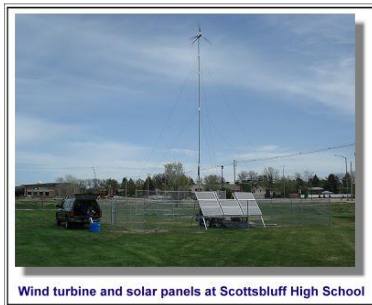
Alternative Energy – The wind and sun power the NDEQ air quality monitoring station in Scottsbluff, NE. Courtesy, Scottsbluff Star Herald
