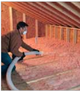
Installing attic insulation during a home weatherization project
