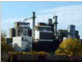
Sheldon power plant near Lincoln
