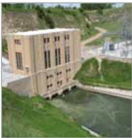
Jeffrey, Johnson 1 Hydroelectric plant southeast of Lexington
