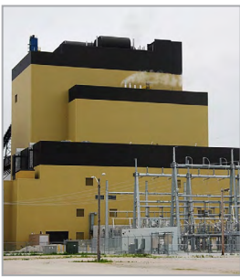
Whelan Energy Center Unit No. 2 in Hastings, Nebraska
