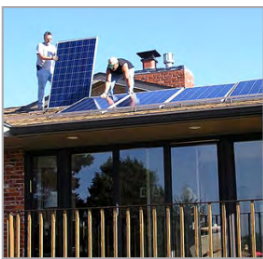
Workers install solar panels atop a home in Lincoln, Nebraska.
